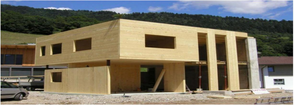
**Smart Green House (SGH)** is a unique integration of the latest developments in the field of wood processing and pre-cut construction method. Compliance with the environmental standards BREEM (Great Britain) and LEED (USA).
